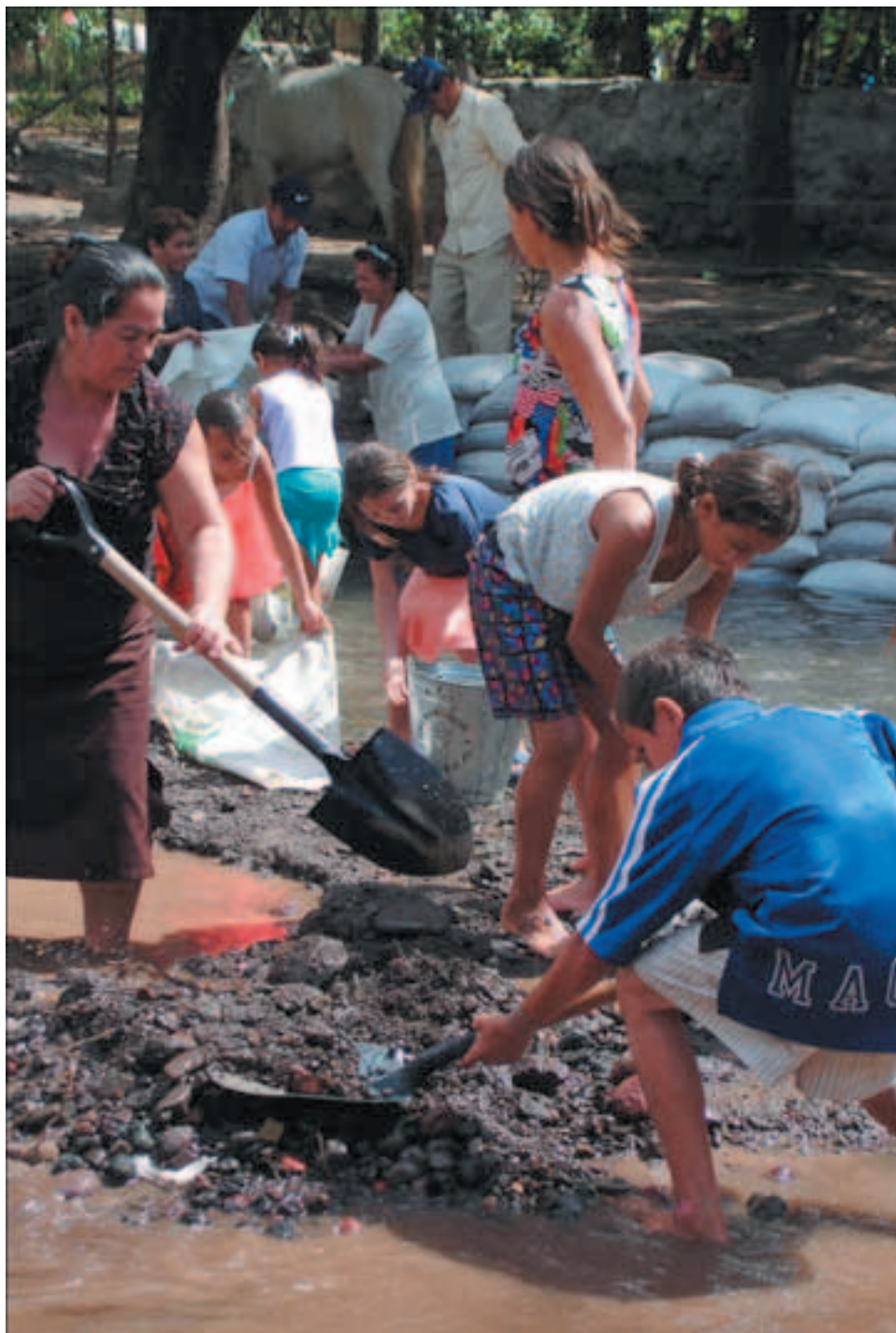
Flooding is a major problem for the people of El Molino Sur in Matagalpa, central Nicaragua. Here they are building up the local river bank, to protect their homes during the wet season.
