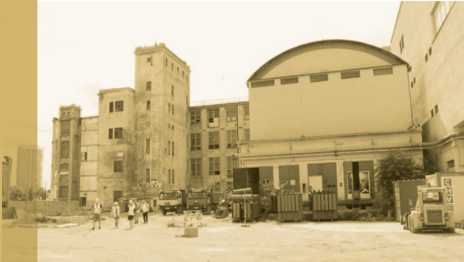
Old Cvernovka building site, on the horizon you see the heritage protected building of the Pradiareň (Spinning Mill), photo: Zdeňka Lammelová
