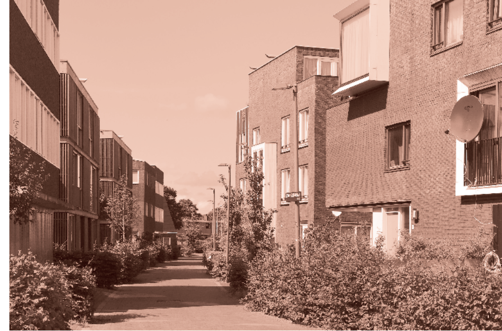
Fig. 7. Reaching for the sustainable density of the Dutch model, Amsterdam, De Bongerd, Rudy Uytenga Architectenbureau, source: UNIT architekti s.r.o.
